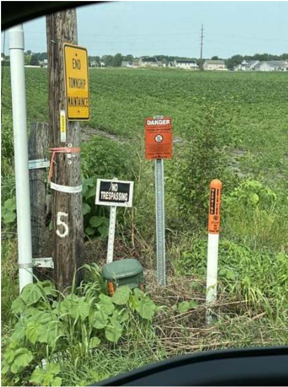
Buried Transport Fiber
